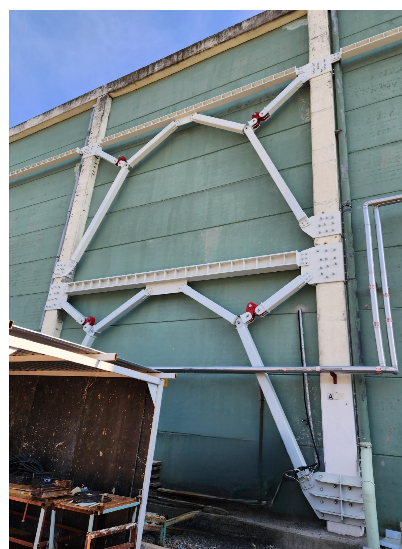
Photo 1: Installed Friction Dampers, Application from Outside.
