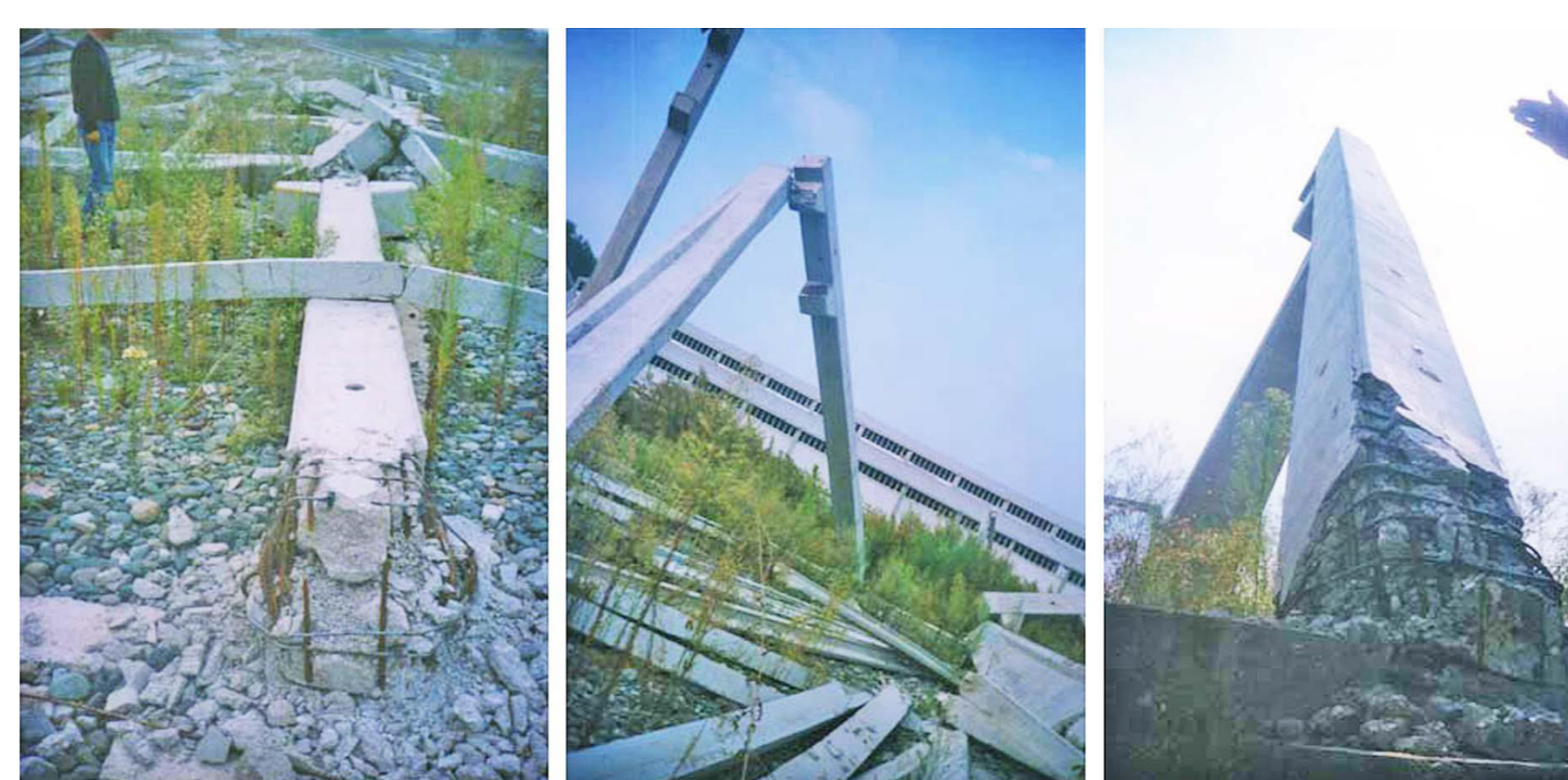
1999 Kocaeli Earthquake Prefabricated Building Damage K.A.Korkmaz, A.E.Karahan June 2011
