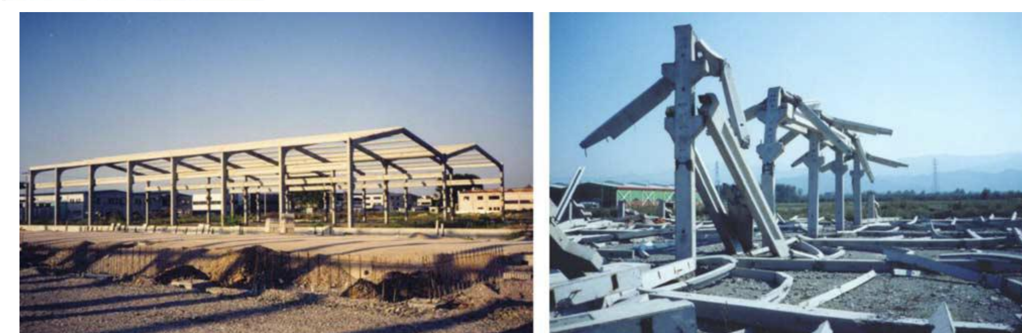
1999 Kocaeli Earthquake Prefabricated Building Damage M.H.Arslan, H.H.Korkmaz, F.G.Gulay December 2004
