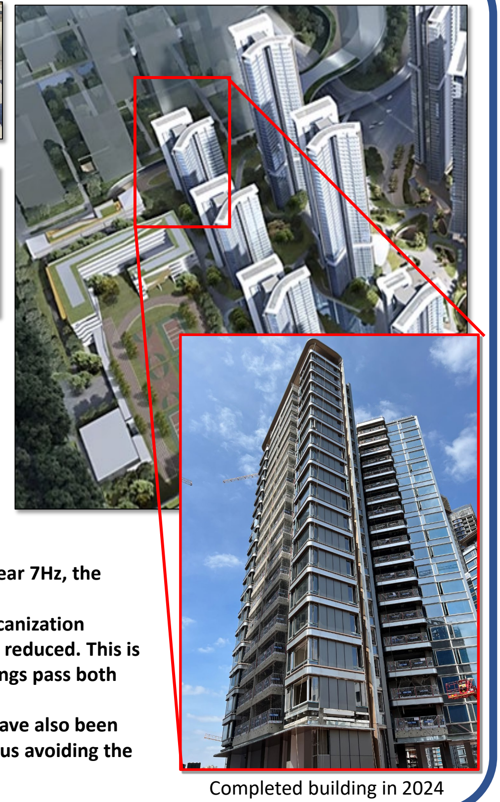
Completed building in 2024
