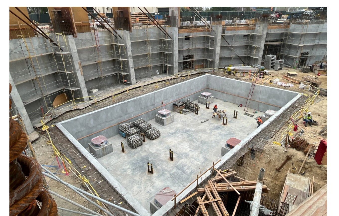
Reinforced concrete pit with isolators placed on site
