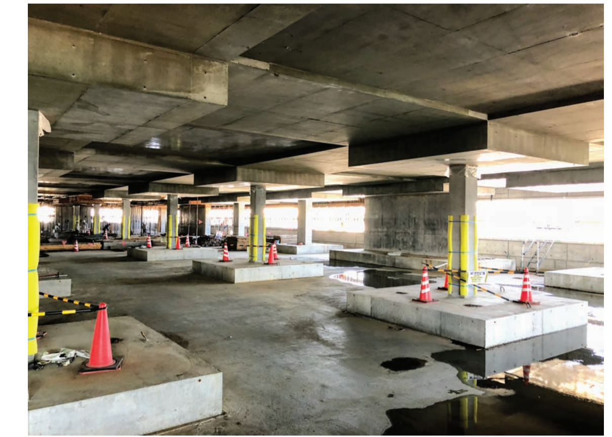
Fig.5 Flat slab with inverted capital
