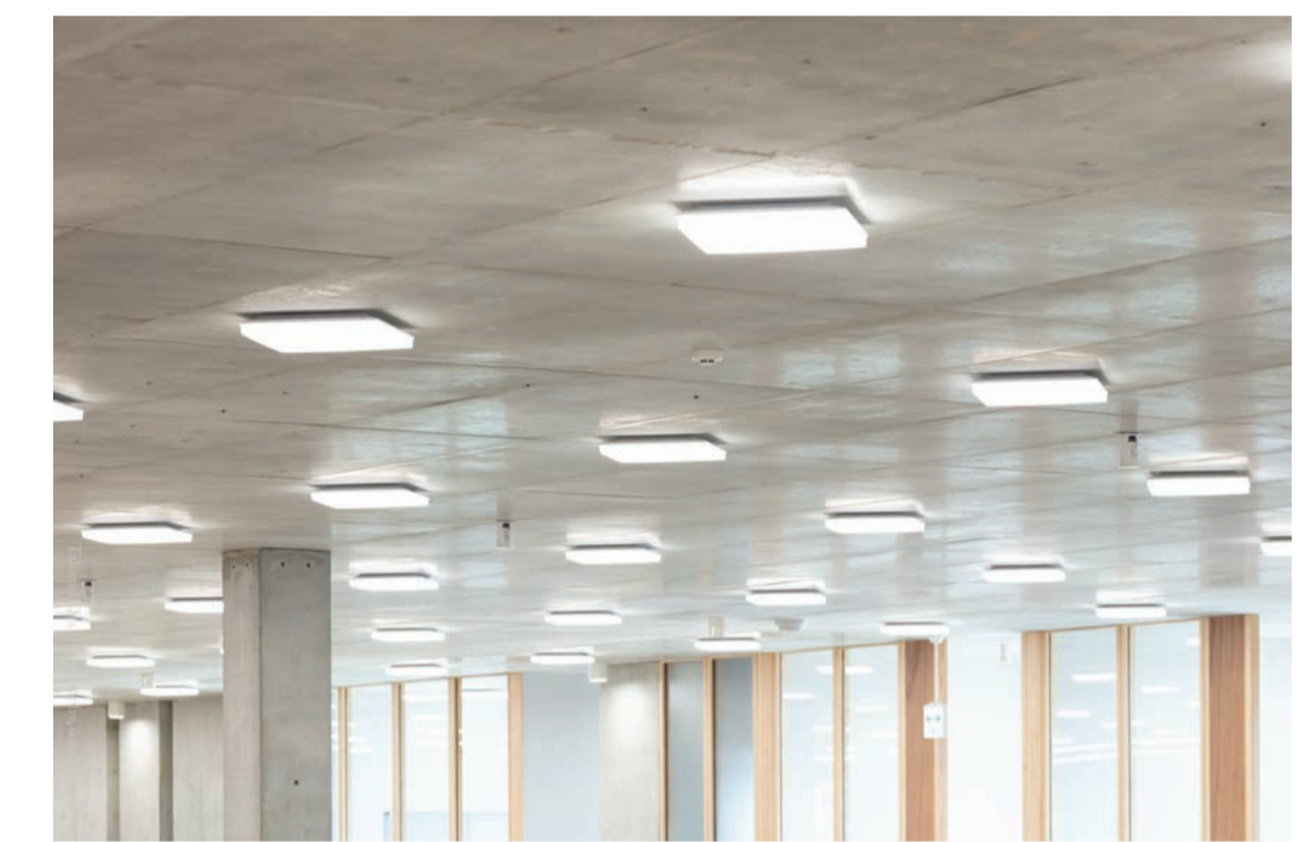
Fig. 6 Interior view of first-floor ceiling without ceiling material
