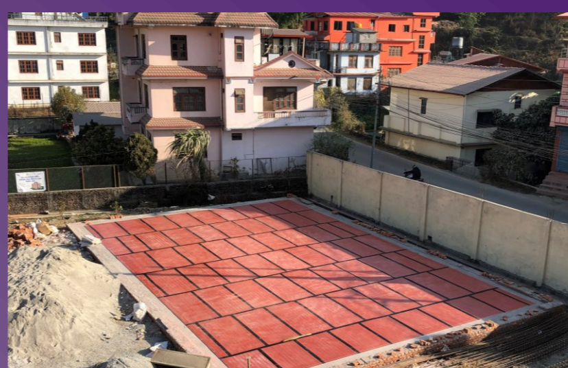
Laying of Upper PVC layer
