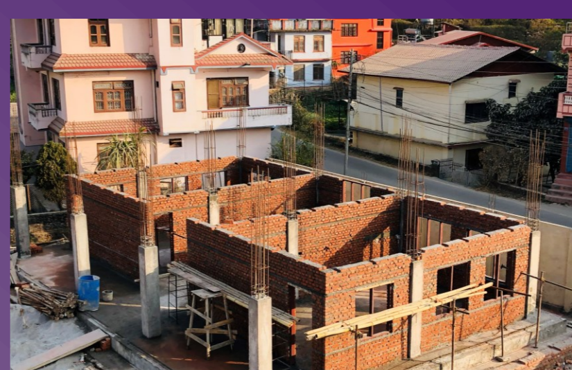
Brickwork completion
