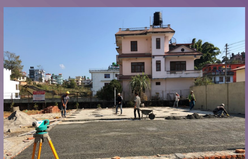
Preparation of the base
