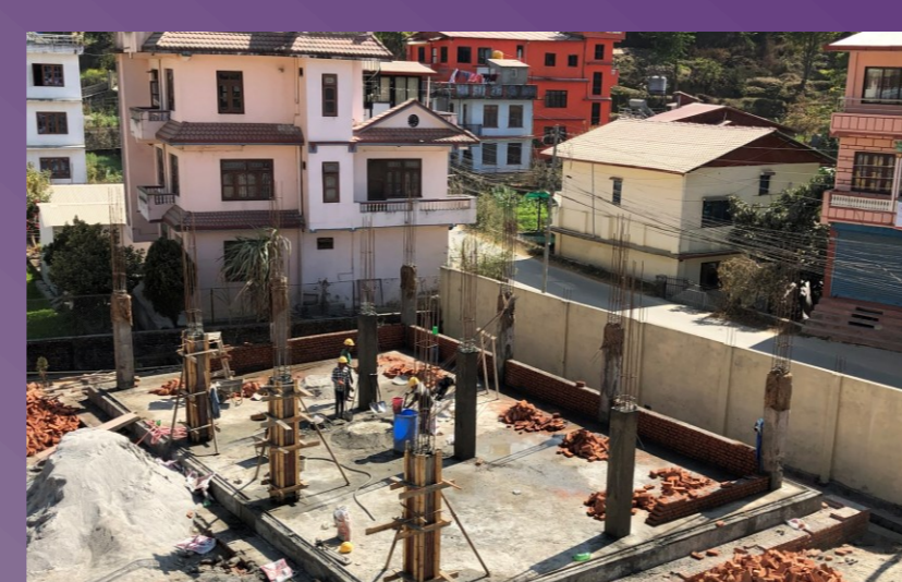
Column concreting
