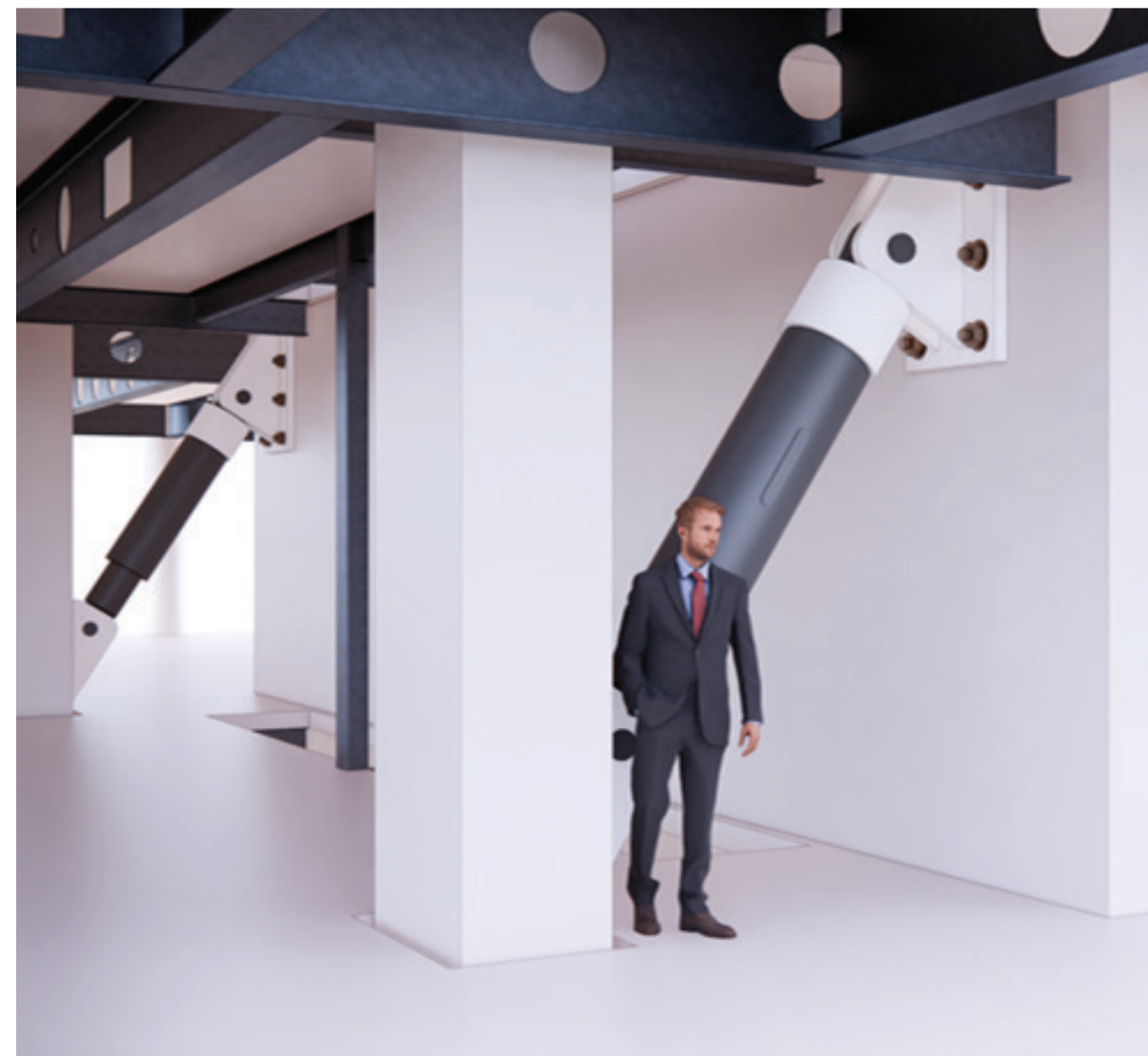
Minimised Obstruction due to tuned Fluid Viscous dampers
