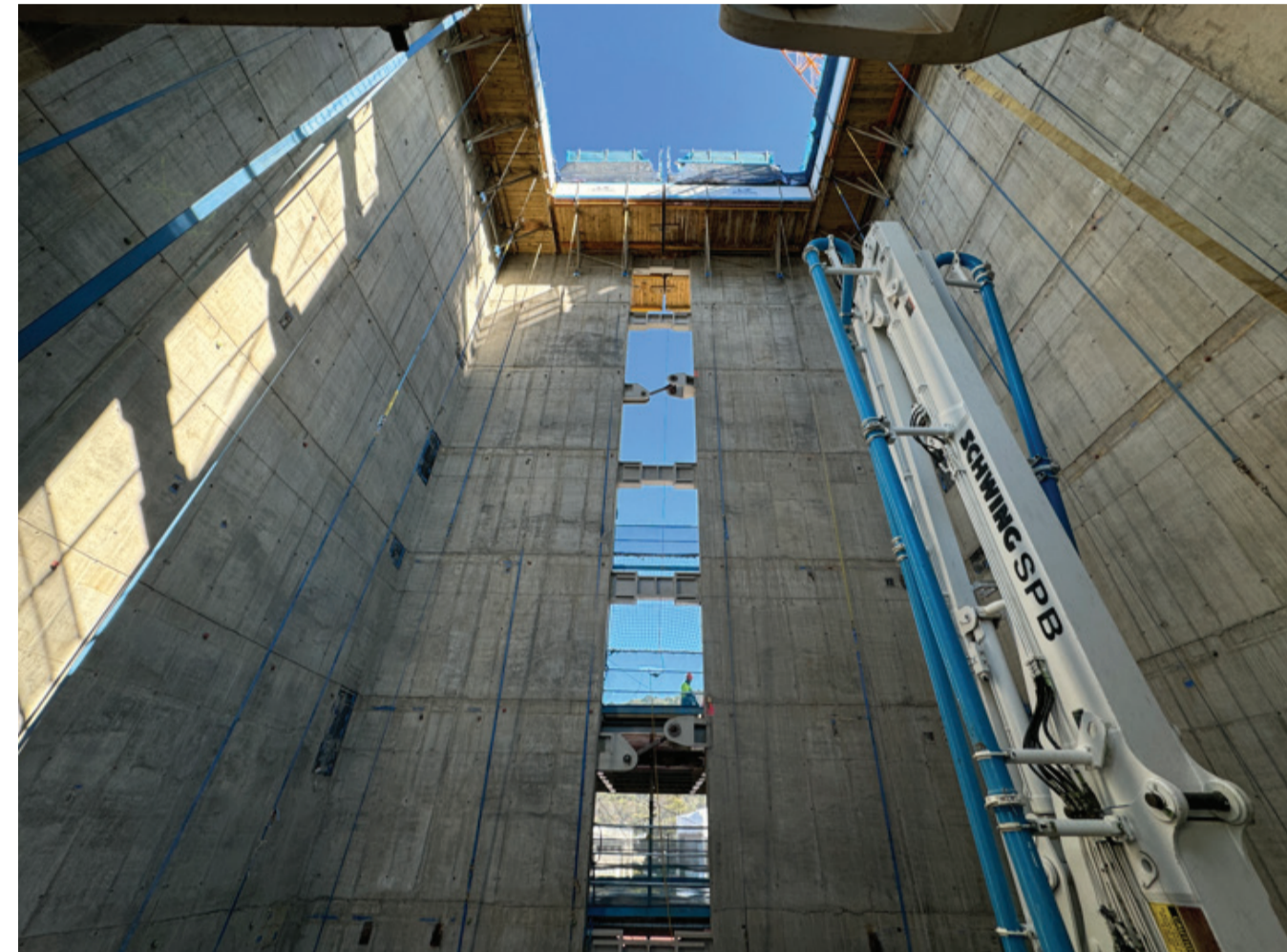
Core wall during construction
